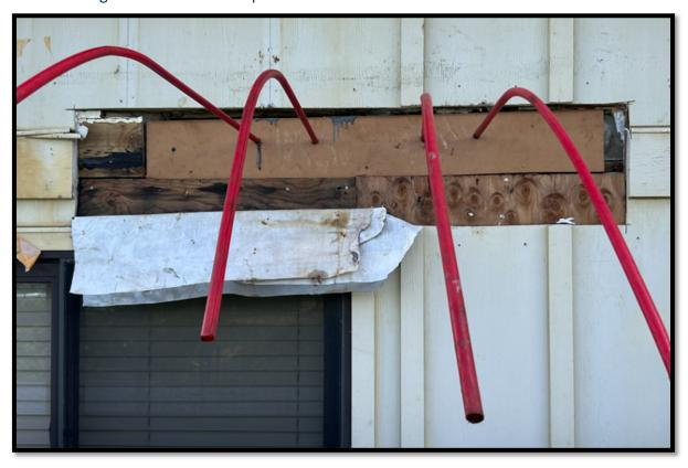
New couplers in front of temporary lock-offs with new end cables in red sheathing
