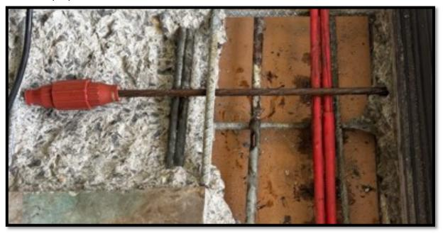
• Ends of 4 new full-length (~200') PT cables with end anchors and sheathing at G22 slab edge
