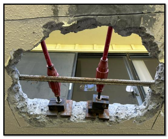
• New transverse cable ends in sheathing from couplers in front of temporary lock-offs on G22 lanai . . . .
