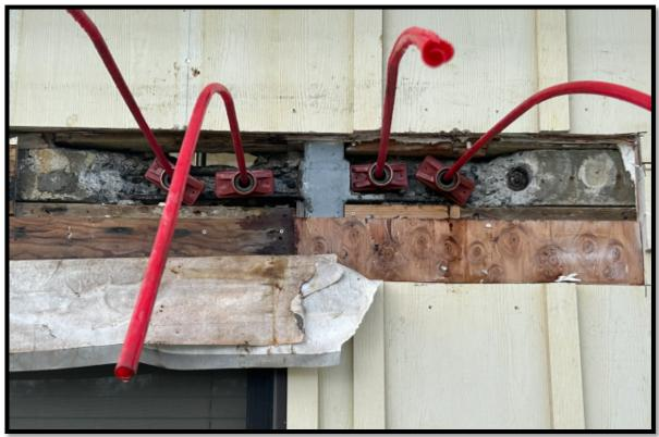
• Slab edge form for concrete patch behind and in front of end anchors
